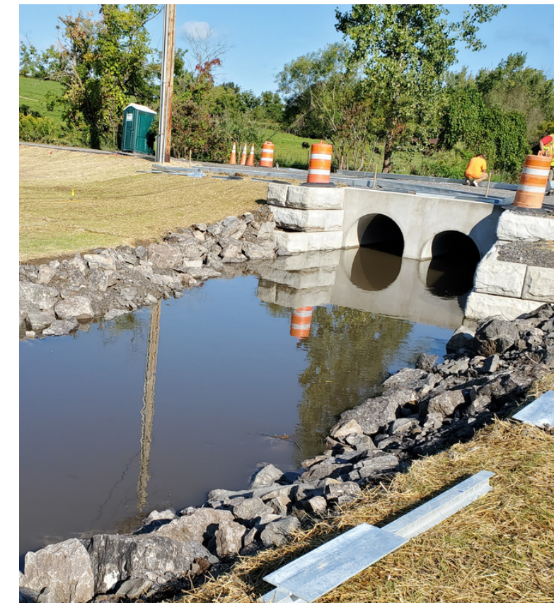
ALDRICH ROAD DRAINAGE PROJECT
