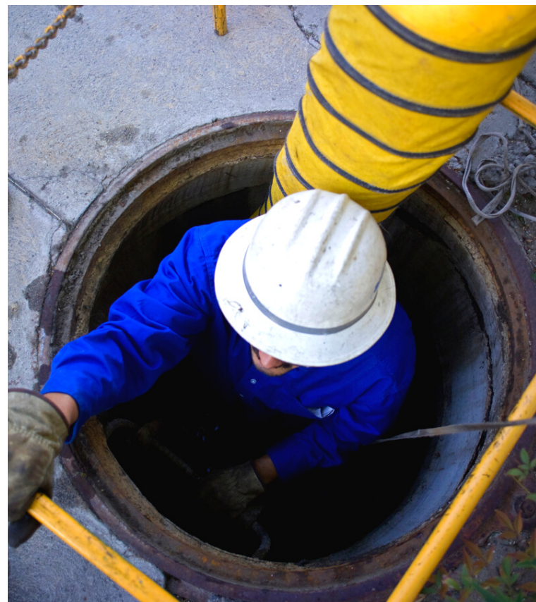
LINED 2,567 LFT OF STORM SEWER, 727 LFT OF SANITARY SEWER
