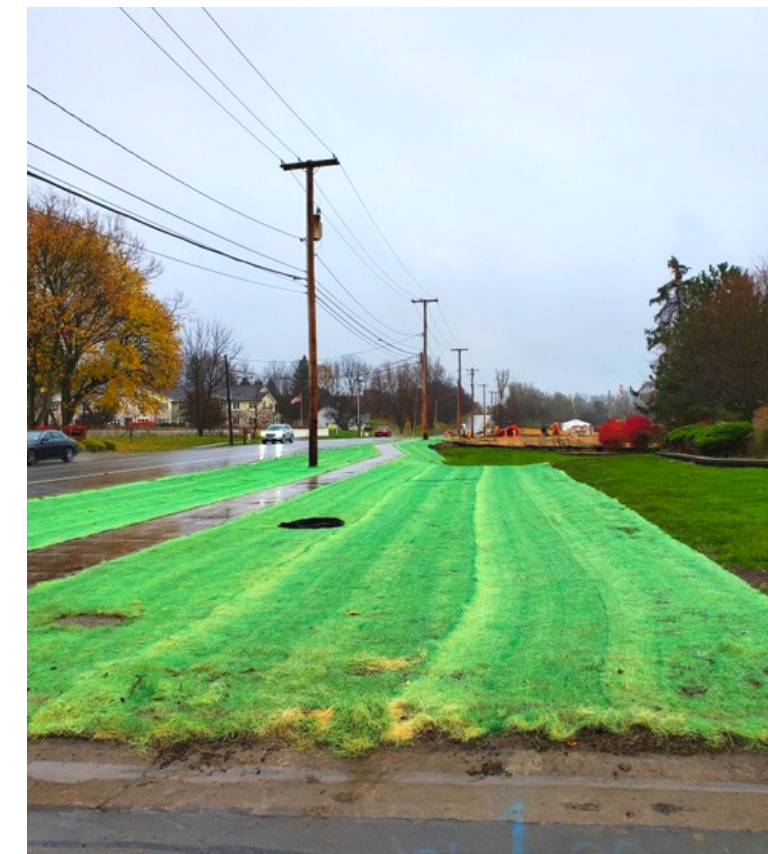
EAGLESFIELD WAY SIDEWALK/DRAINAGE IMPROVEMENTS
