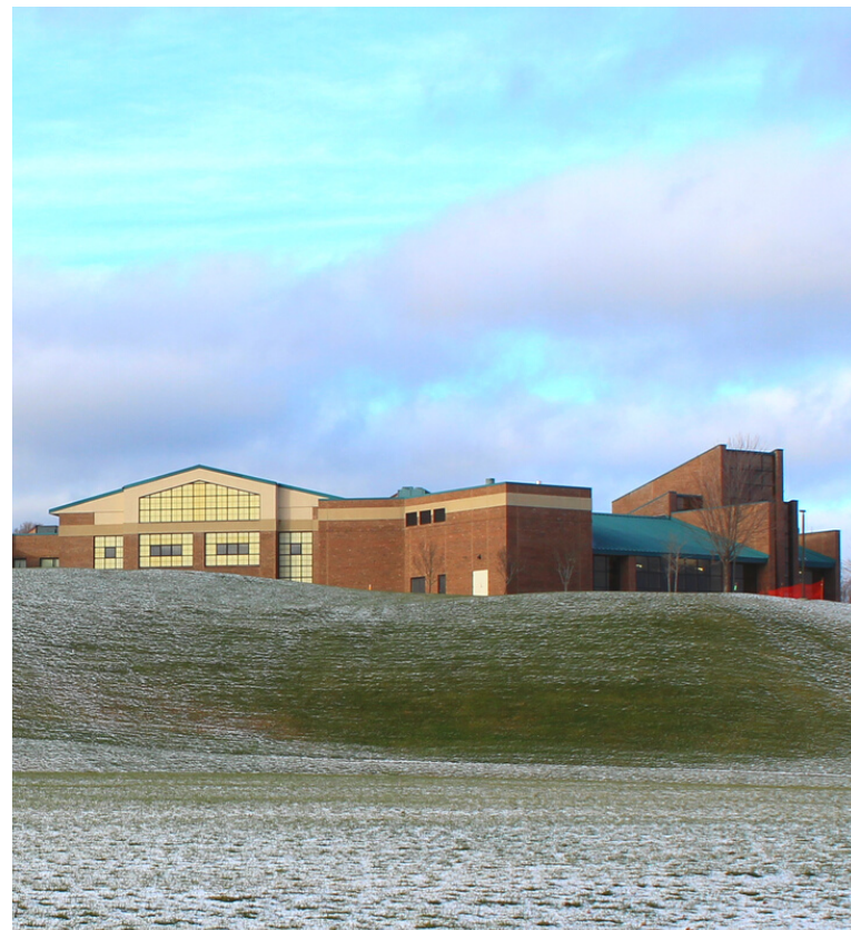
PCC LIGHTING ASSESSMENT; SECURING 100K LED GRANT
