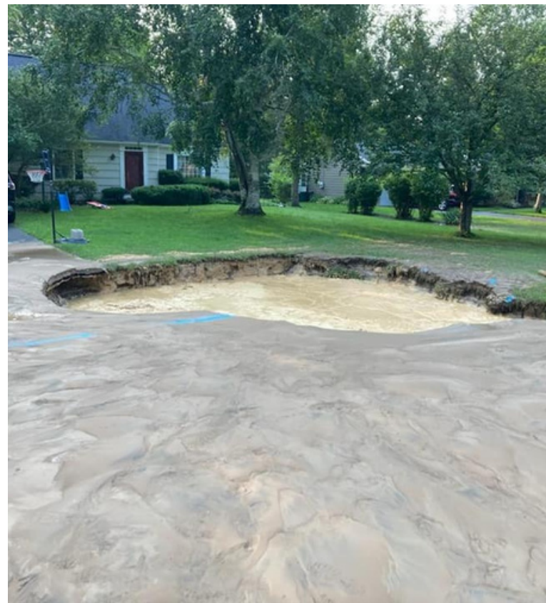
EMERGENCY CLEAN-UPS FROM WIND/FLOODING
