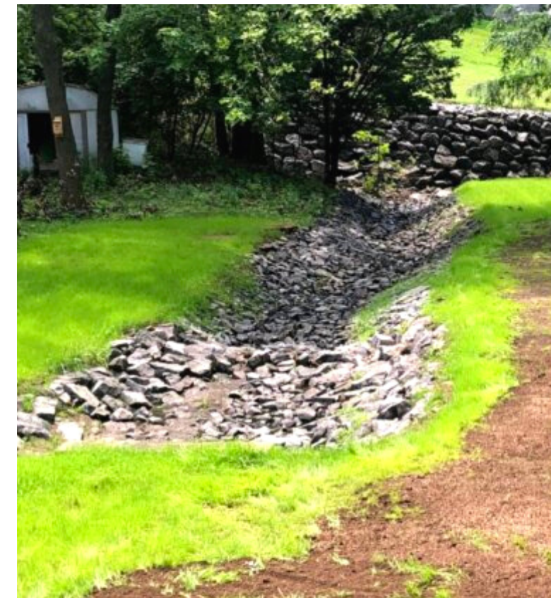
OLD POST STREAM BANK STABILIZATION
