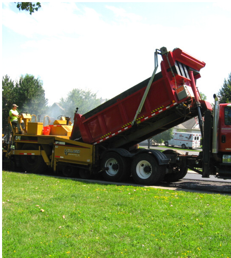
ROAD REHABILITATION: 4.5 MILES OF MILL/ PAVE, 21 MILES OF CHIP SEAL
